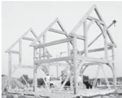
Raising the white oak frame in Oskaloosa, Kansas, Workshop, June 2002
