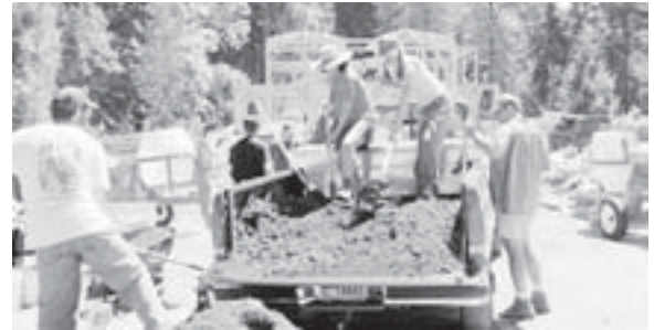
Clay was harvested from the side of the drive into the site.
