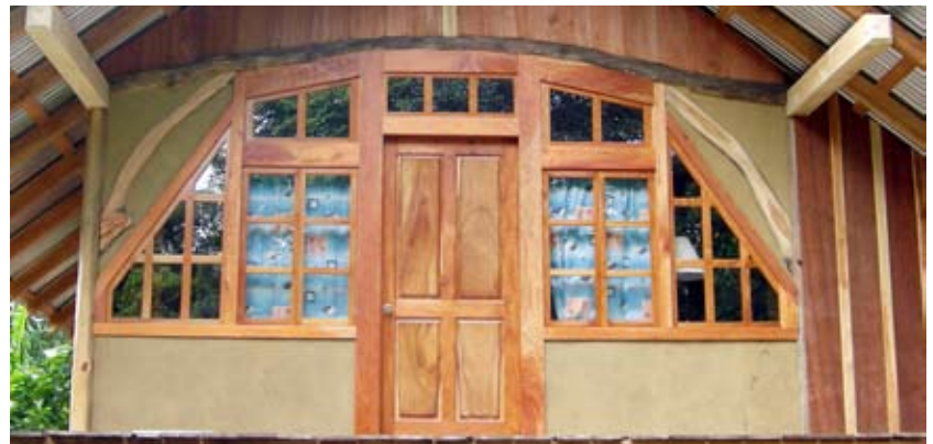
Completed wall system using wattle & daub and clay plaster.
