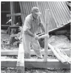
Finca la Bella community elder splitting bamboo wattles. Bamboo, a plentiful resource in Costa Rica, can be used for numerous building applications, from structural members; purlins and common rafters. to roofing.
